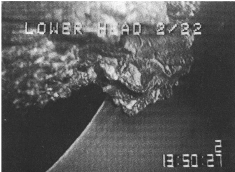
Figure 20. Lumps of agglomerated material that appeared to have been molten, congealed, and then broken off inside the hole.
